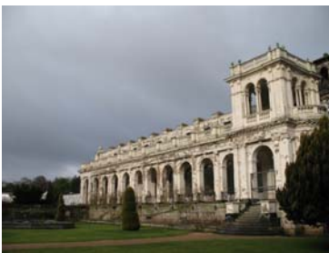
South Elevation of Former Service Block
