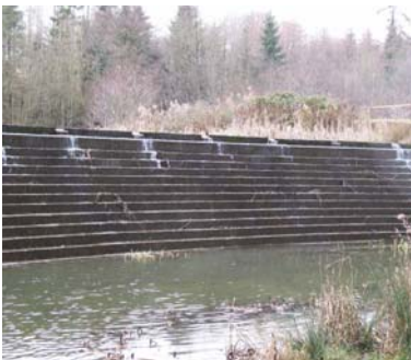
Stone weir on Lake shore
