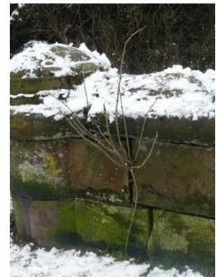
Condition of Bridge
