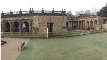
Grand Entrance in Poor Condition
