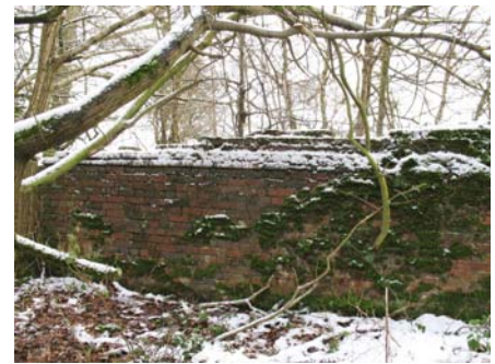
Part of Boundary Wall
