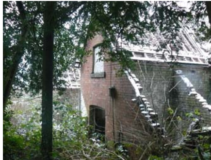
1-4 Park Drive, a Derelict Listed Building
