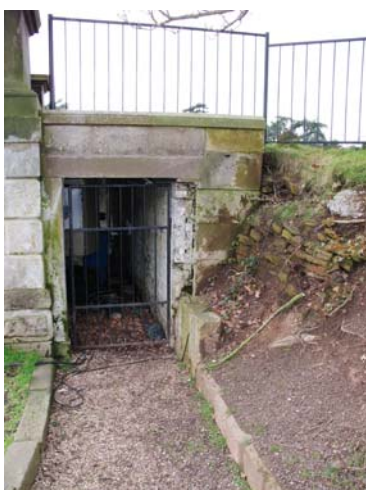
Damage to Side Entrance of Boathouse
