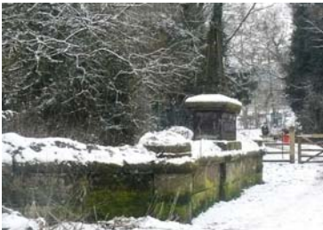
Eighteenth Century Single-span Bridge
