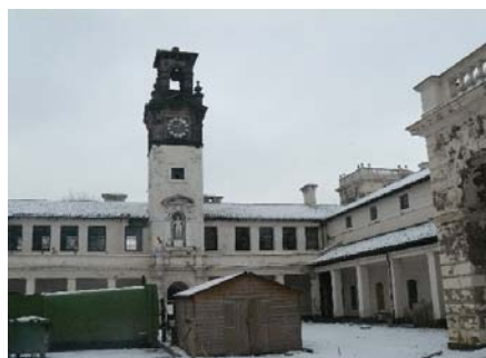
Rear Courtyard in Poor Condition
